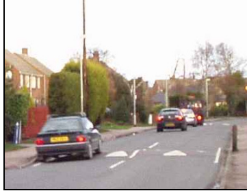
Fig. 2. Photo of speeding traffic crossing a speed hump, swerving curbside to minimize bump.
